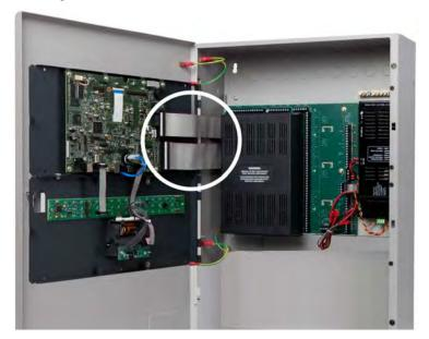
Remove four hinge-pins of the Fascia and then remove the Fascia from the Cabinet-Box of the FACP. 6 Return the four hinge-pins to the hinges of the Cabinet-Box for safekeeping.
